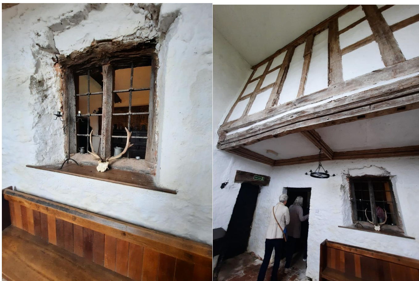
Iron grill through which servants would view the service, and above the now filled-in gallery from where the ladies of the family would view the service.
