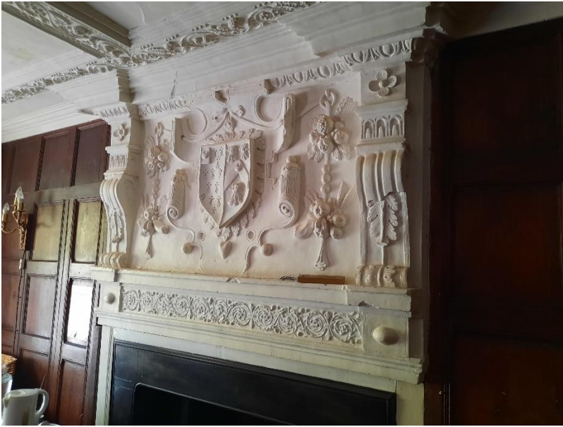
The room above the small dining room, built at the same time as the room below, with similar motifs in the plasterwork.
